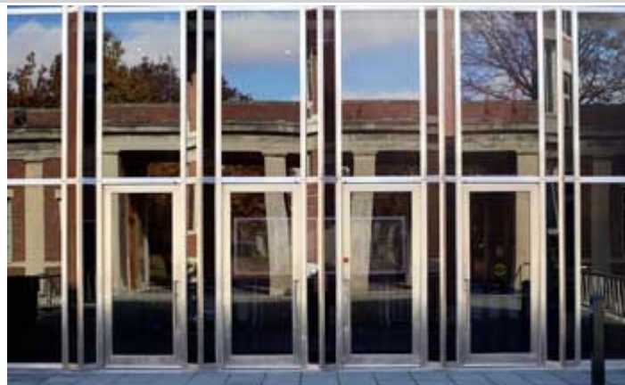
Entrance to Hoyt
